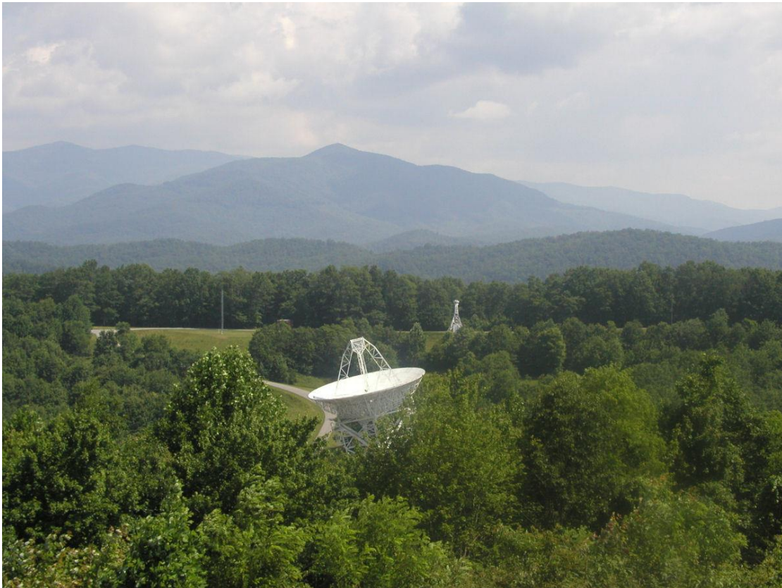
Fig. 5. Concave Radio Telescope Dish with Receiver at the Focal Point.
