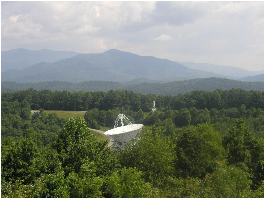
Fig. 5. Concave Radio Telescope Dish with Receiver at the Focal Point. Photo by Doc, June 13, 2002, at PARI, Rosman, NC
